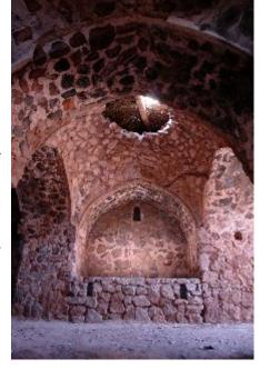
suburb of a village of the same name. Robat of Qarabil is made of stone and mortar and has a rectangular plan with a large portal on the south wall. The Robat has two courtyards both open to the sky and the inside walls of the enclosure is outfitted with a number of identical niches or chambers to accommodate merchants and their servants, animals, and merchandise.
